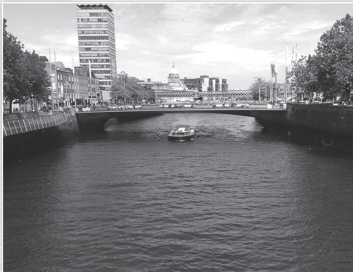
THE ROSIE HACKETT BRIDGE IN DUBLIN.
