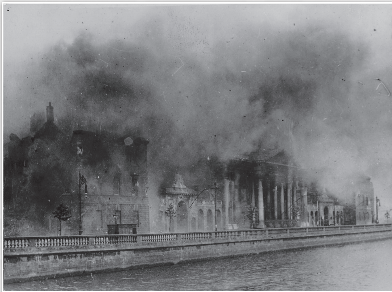
THE FOUR COURTS ON FIRE.
