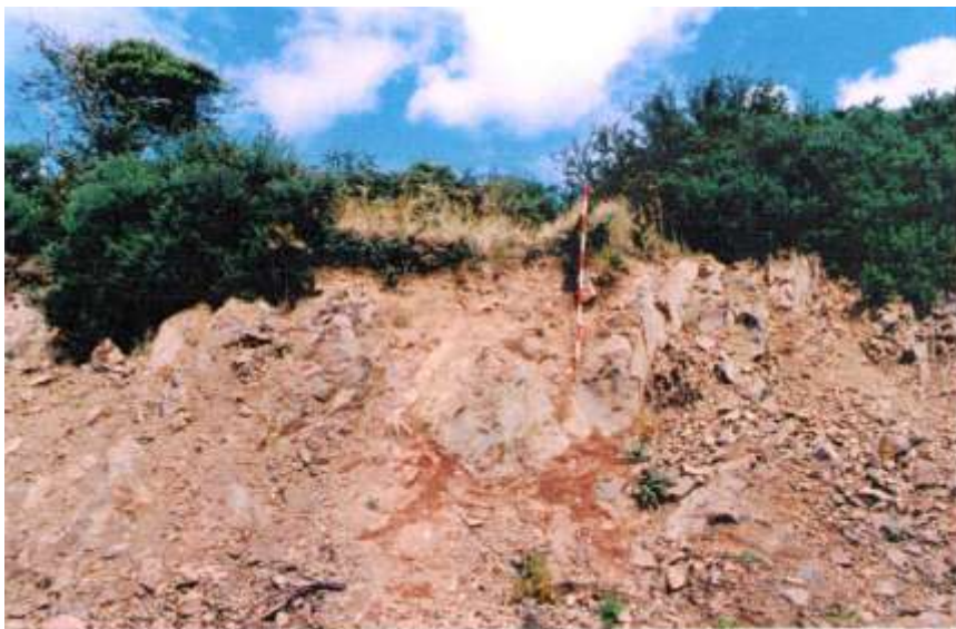
Figure 50: Section of ditch in the north face of Ardkill More quarry (Campbell 1997, photograph 2) (courtesy: Kieran Campbell).
