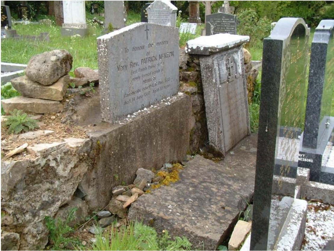
Old Foundation of Building
