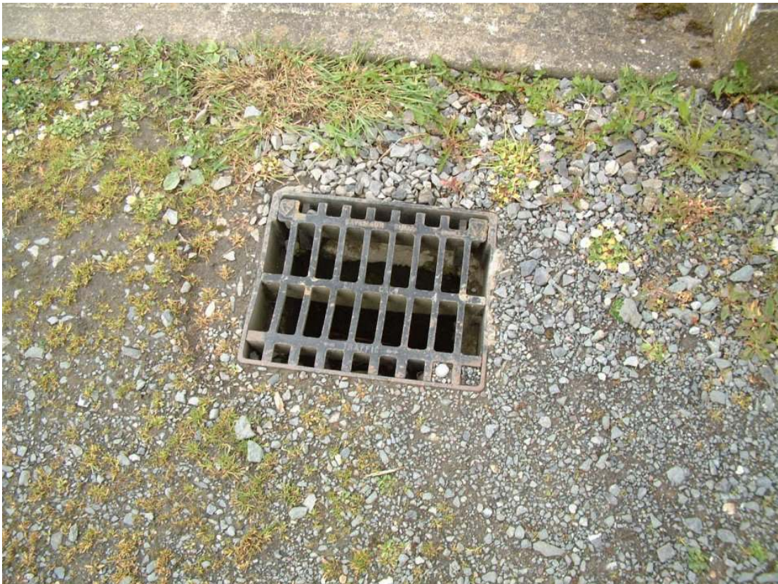
Part of Drainage System
